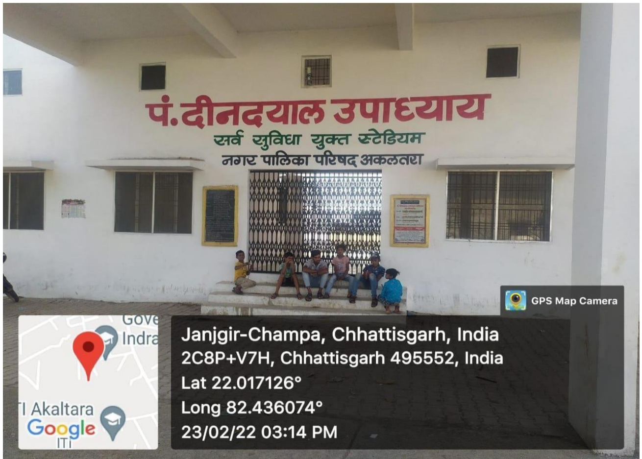
Indoor Outdoor Stadium (Municipal Corporation Akaltara)
